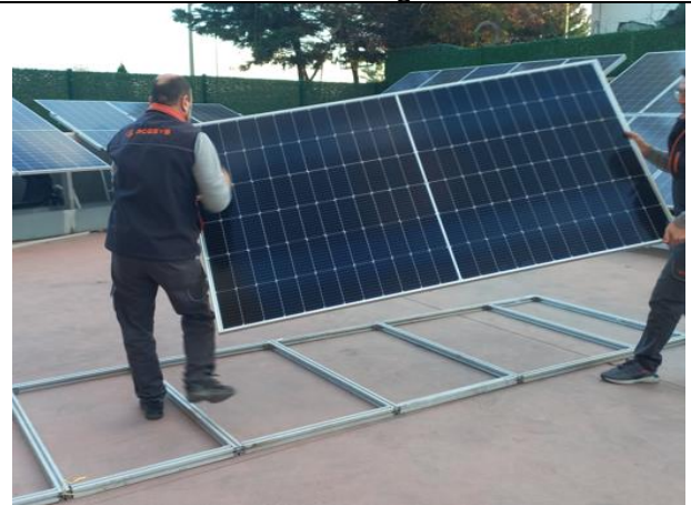
Photo 22: Installation and Dismantling of the Panels
